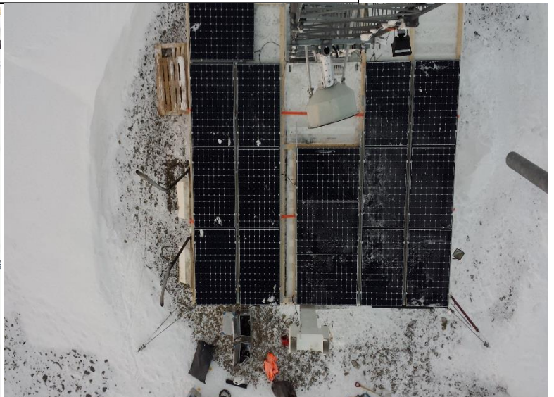
Fig 1 – paneler tak (horisontal montering)
