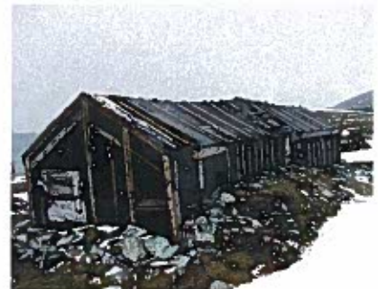
A trappers hut with a thick layer of turf for insulation purposes. This keeps the water content high inside the walls
